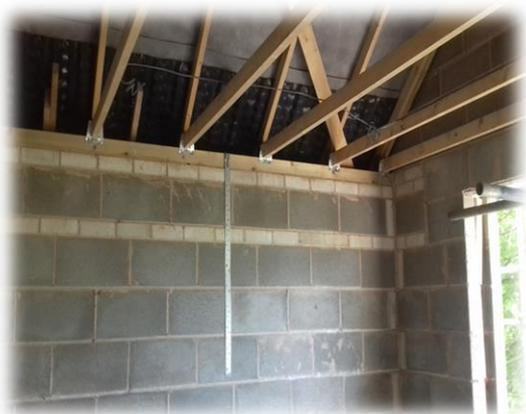
*Fig 4* incorrectly installed eave vent tray
